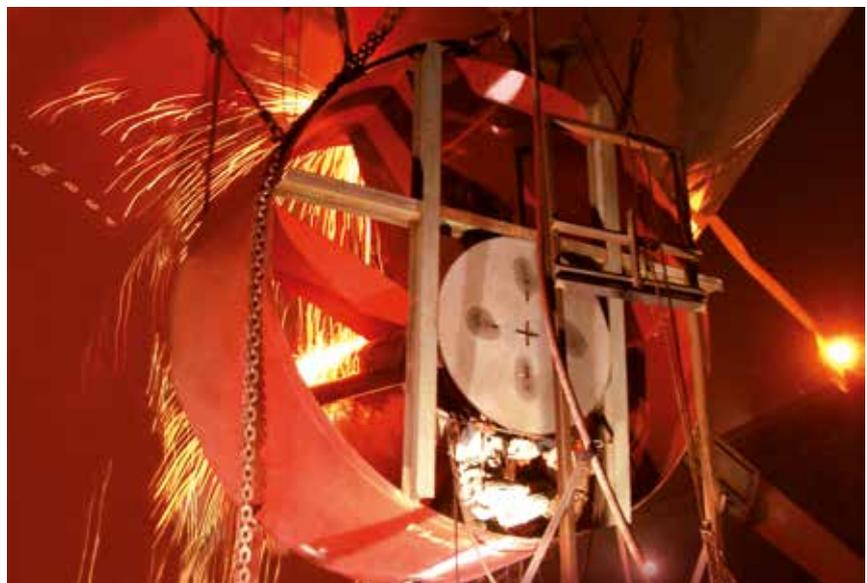
FIGURE 1 - The installation of a Becker Mewis Duct®
